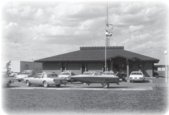
Pictured is Sikeston Satellite Station, which opened October 1, 1973.
